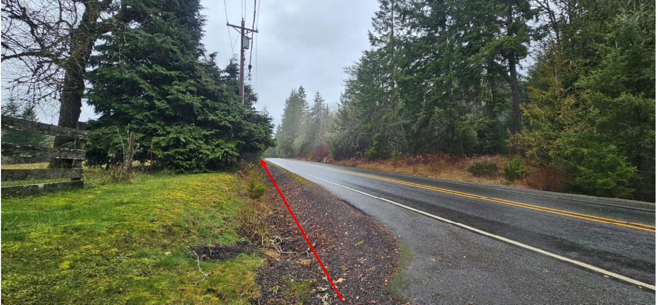
Figure 2 A– Site Access on Highway 47 (Looking South ~ 385 Feet Line of Site)
