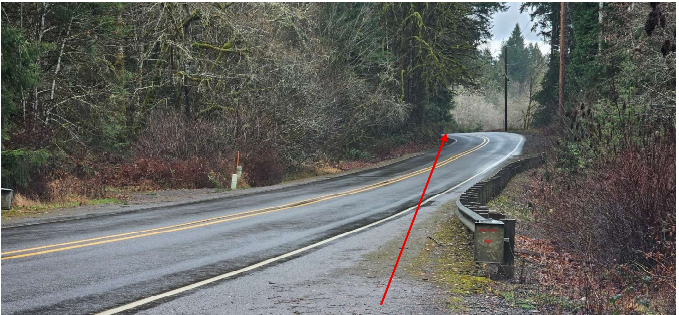
Figure 2 B– Site Access on Hwy 47 Looking North – Over 520 Feet Line of Site
